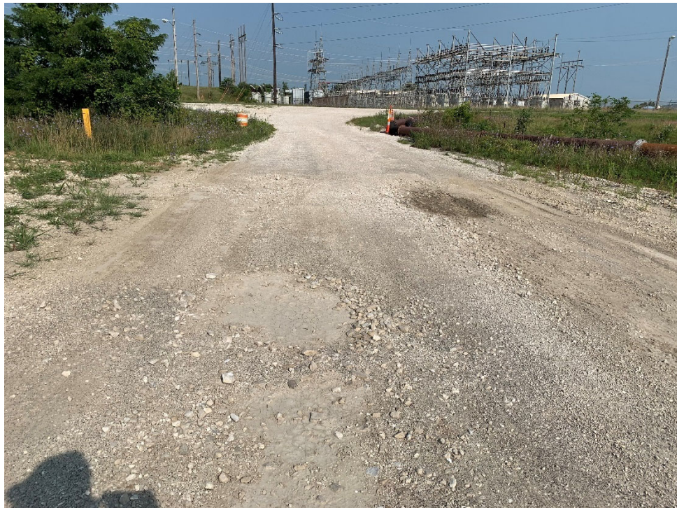
Photo No. 22 Aggregate road rutting and potholes
