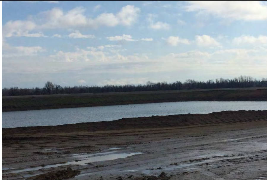
Photograph No. 11 AECI UWL Inspection Sedimentation pond
