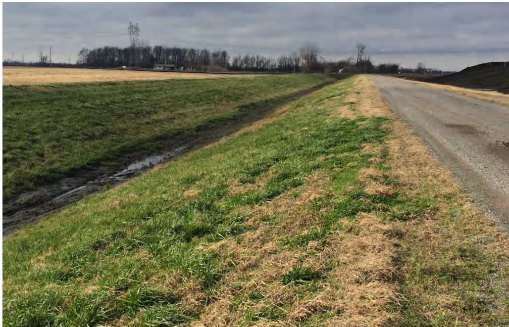
Photograph No. 8 AECI UWL Inspection Stormwater drainage ditch
