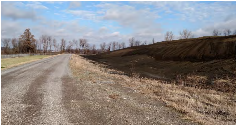
Photograph No. 4 AECI UWL Inspection Western landfill face and perimeter berm/road
