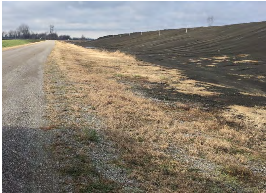
Photograph No. 6 AECI UWL Inspection Southern landfill face and perimeter berm/road
