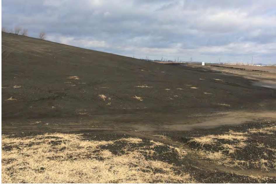
Photograph No. 7 AECI UWL Inspection Eastern landfill face
