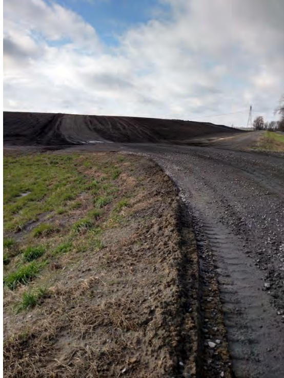
Photograph No. 1 AECI UWL Inspection Haul road approaching northeast landfill corner
