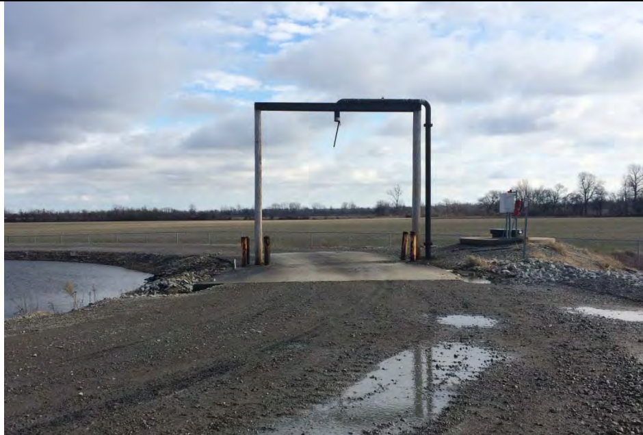
Photograph No. 15 AECI UWL Inspection Leachate loadout structure
