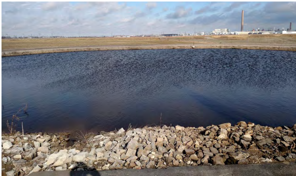
Photograph No. 14 AECI UWL Inspection Leachate collection pond
