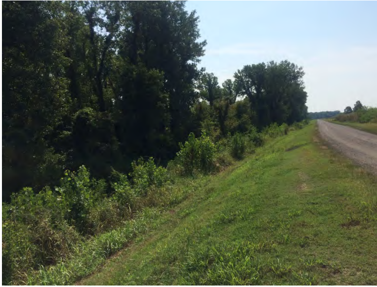
Photograph No. 3 Pond 003 Downstream slope on eastern embankment
