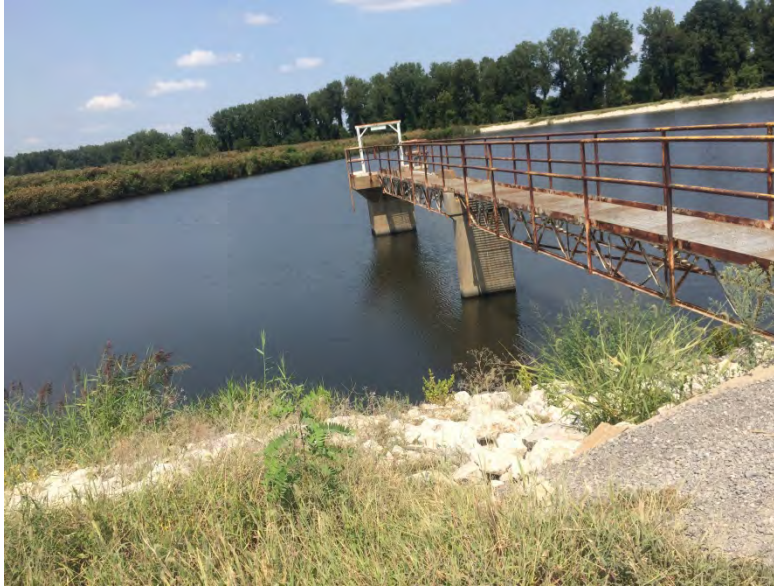
Photograph No. 9 Pond 003 Concrete drop inlet spillway with concrete stop logs
