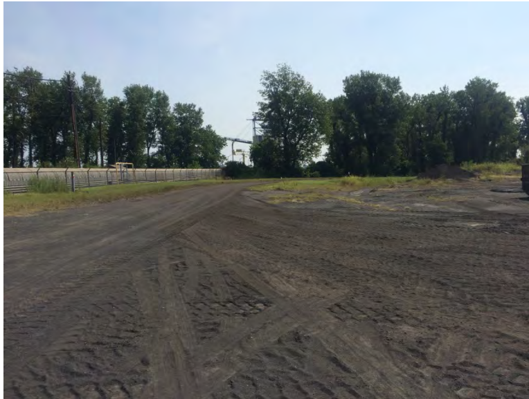
Photograph No. 2 Pond 003 Crest and access road on northern embankment
