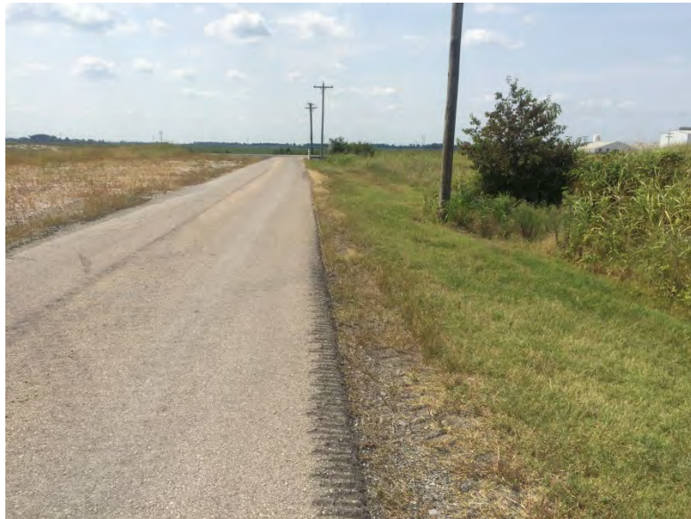
Photograph No. 12 Pond 003 Paved Crest on southern embankment
