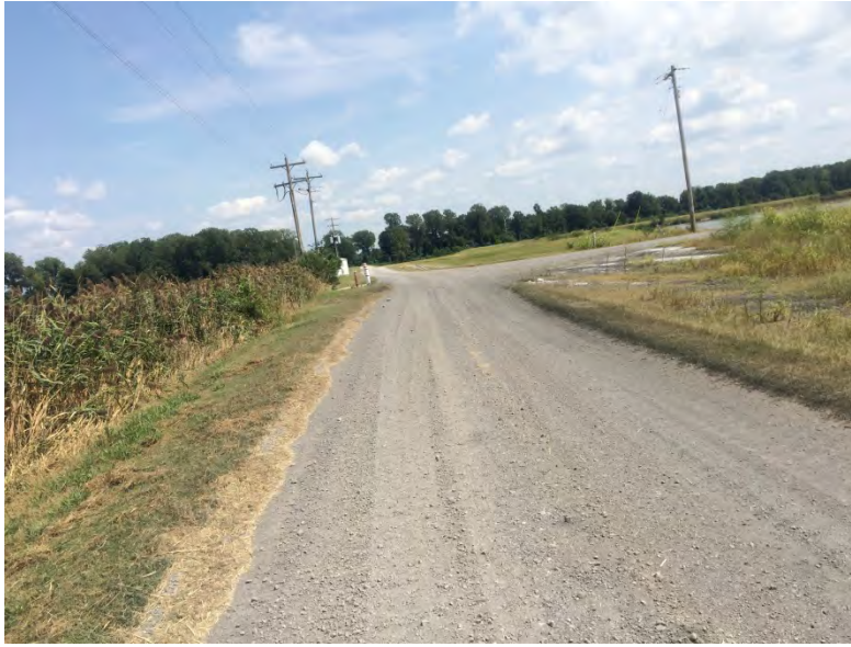
Photograph No. 11 Pond 003 Crest on southern embankment
