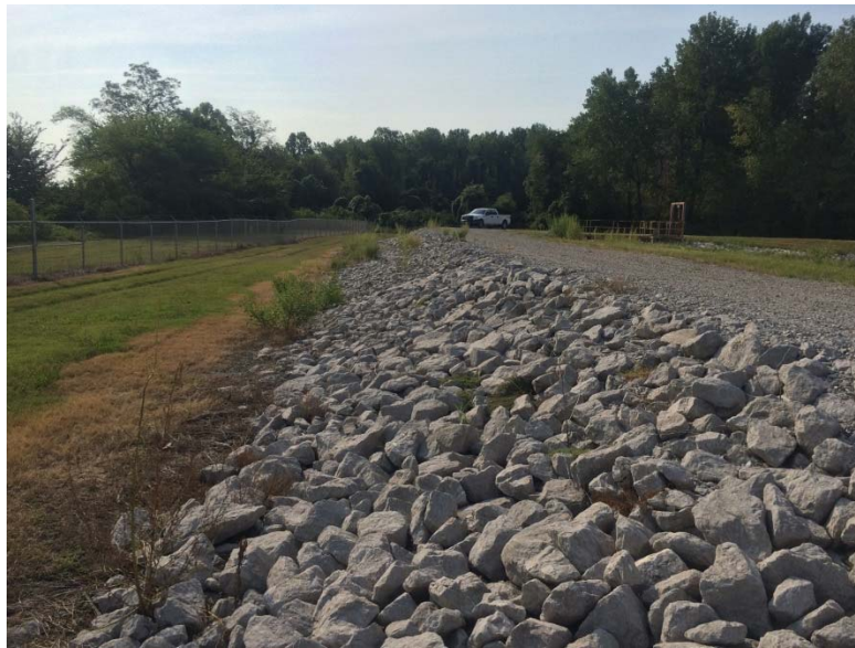
Photograph No. 8 Slag Dewatering Pond Dam (004 Pond) Downstream slope of eastern embankment with riprap
