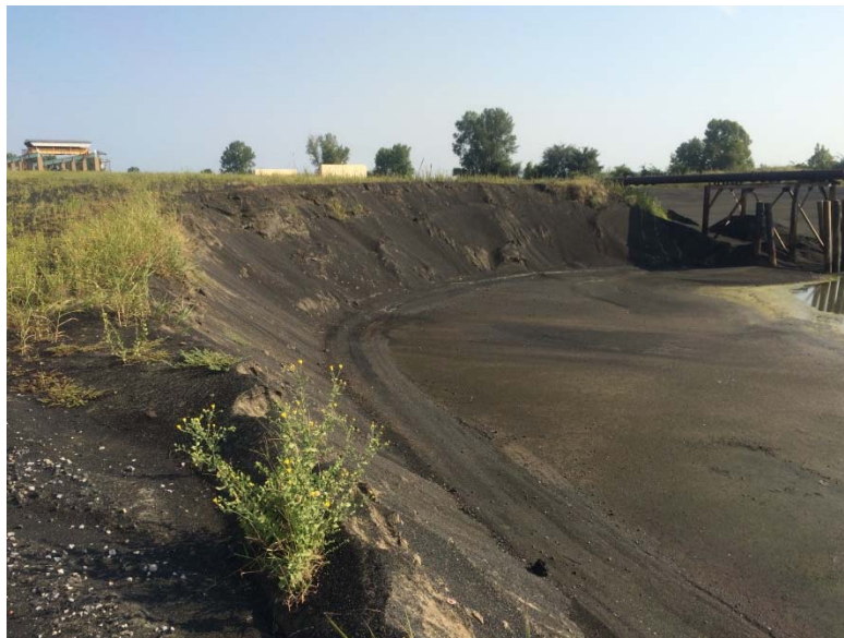
Photograph No. 4 Slag Dewatering Pond Dam (004 Pond) Upstream slope of northern embankment
