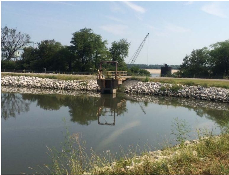
Photograph No. 11 Slag Dewatering Pond Dam (004 Pond) Concrete drop inlet spillway with stoplogs Mississippi River in background
