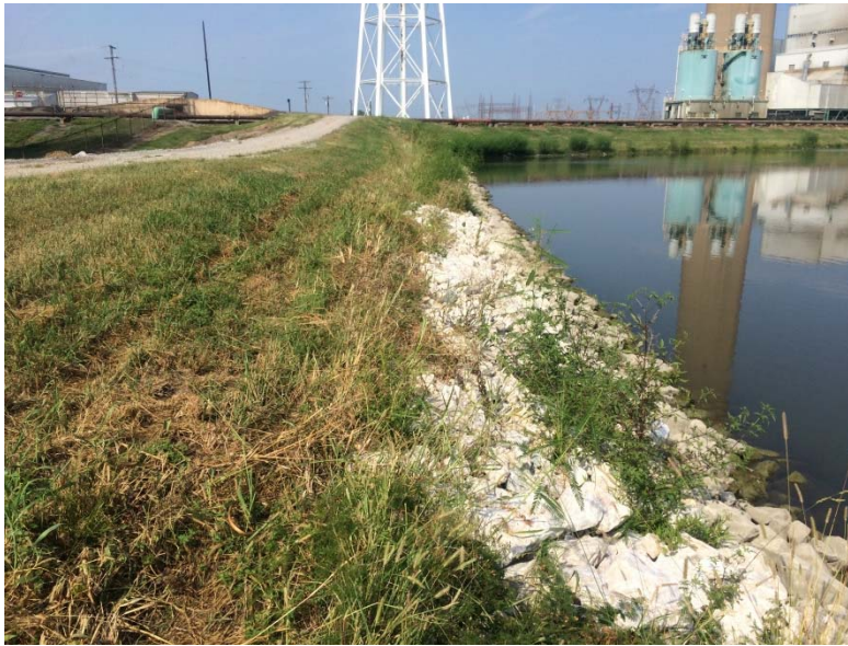
Photograph No. 9 Slag Dewatering Pond Dam (004 Pond) Upstream slope with riprap and vegetation
