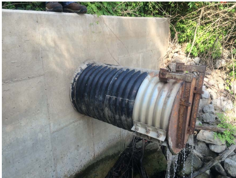
Photograph No. 12 Slag Dewatering Pond Dam (004 Pond) Discharge pipe to Mississippi River with backflow preventer
