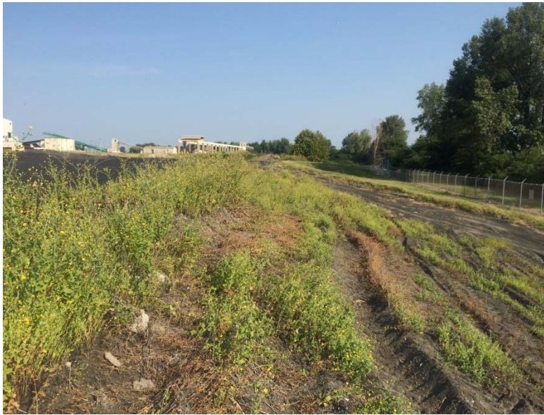
Photograph No. 7 Slag Dewatering Pond Dam (004 Pond) Downstream slope of eastern embankment with ruts and uneven surface
