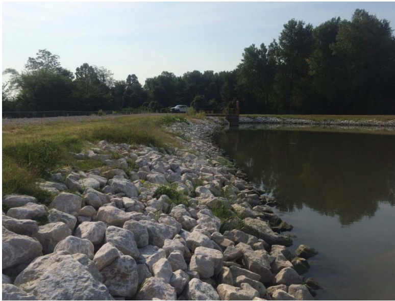
Photograph No. 5 Slag Dewatering Pond Dam (004 Pond) Upstream slope of eastern embankment with riprap and vegetation
