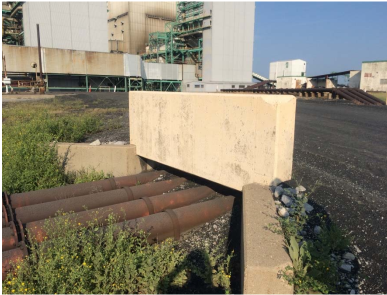
Photograph No. 1 Slag Dewatering Pond Dam (004 Pond) Four inlet pipes with headwall
