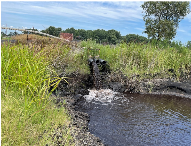
Photograph No. 20 Pond 003 Three inlet pipes interior to unit near northwest corner of unit One pipe (left) actively sluicing
