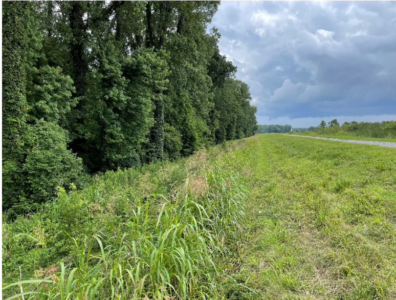
Photograph No. 7 Pond 003 Vegetation on downstream slope of eastern embankment
