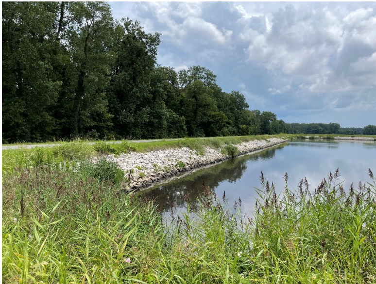
Photograph No. 10 Pond 003 Riprap on upstream slope of southern portion of eastern embankment (ponding area)
