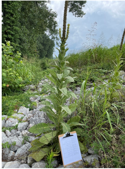
Photograph No. 5 Pond 003 Vegetation in riprap on downstream slope of eastern embankment
