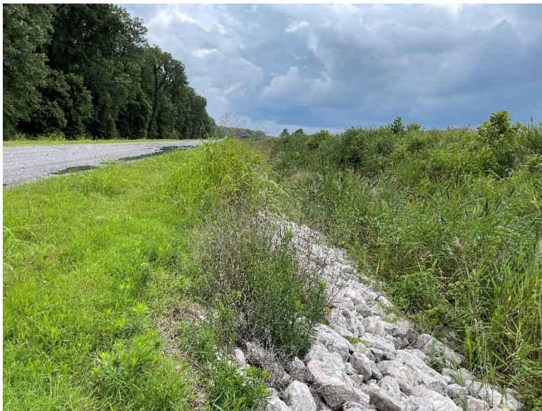
Photograph No. 8 Pond 003 Vegetation and riprap on upstream slope of eastern embankment Interior drainage channel at right
