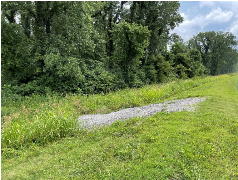
Photograph No. 2 Pond 003 Graveled access point to monitoring wells on downstream slope of eastern embankment
