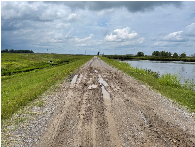
Photograph No. 12 Pond 003 Rutting in crest of eastern portion of southern embankment
