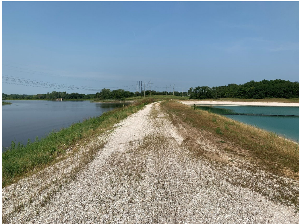
Photo No. 2 Aggregate surface on Cell 002 embankment crest
