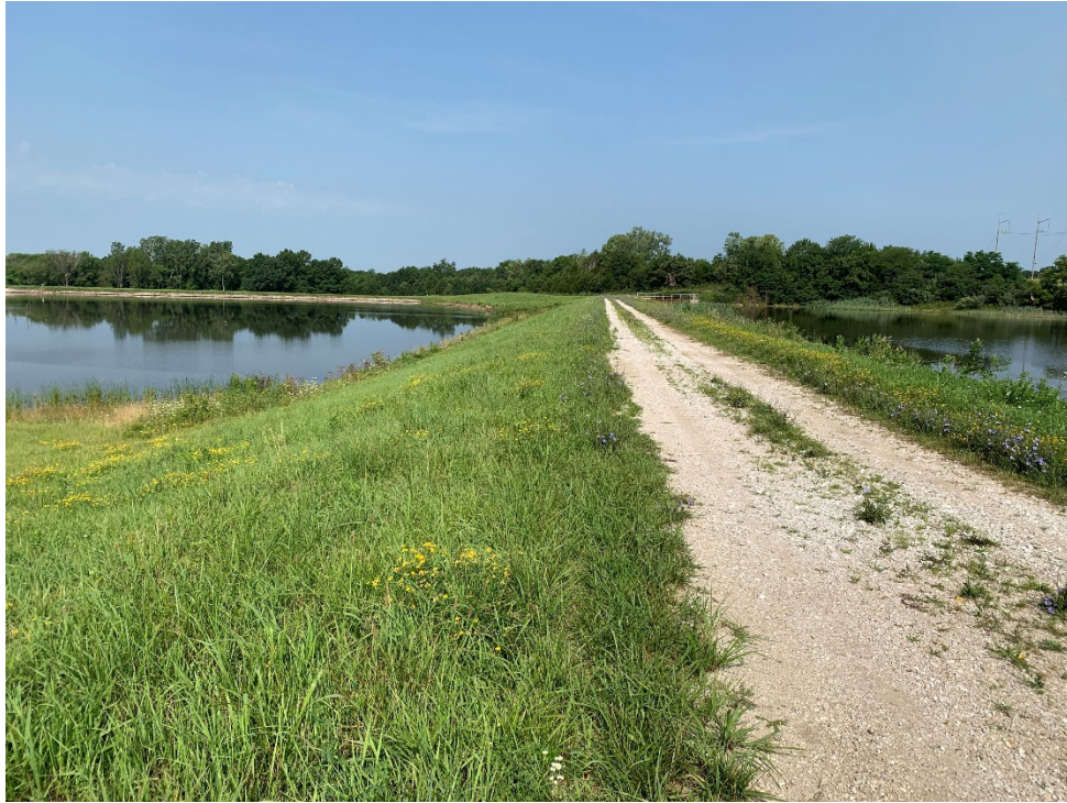
Photo No. 9 Downstream slope and aggregate surface atop Cell 003 embankment
