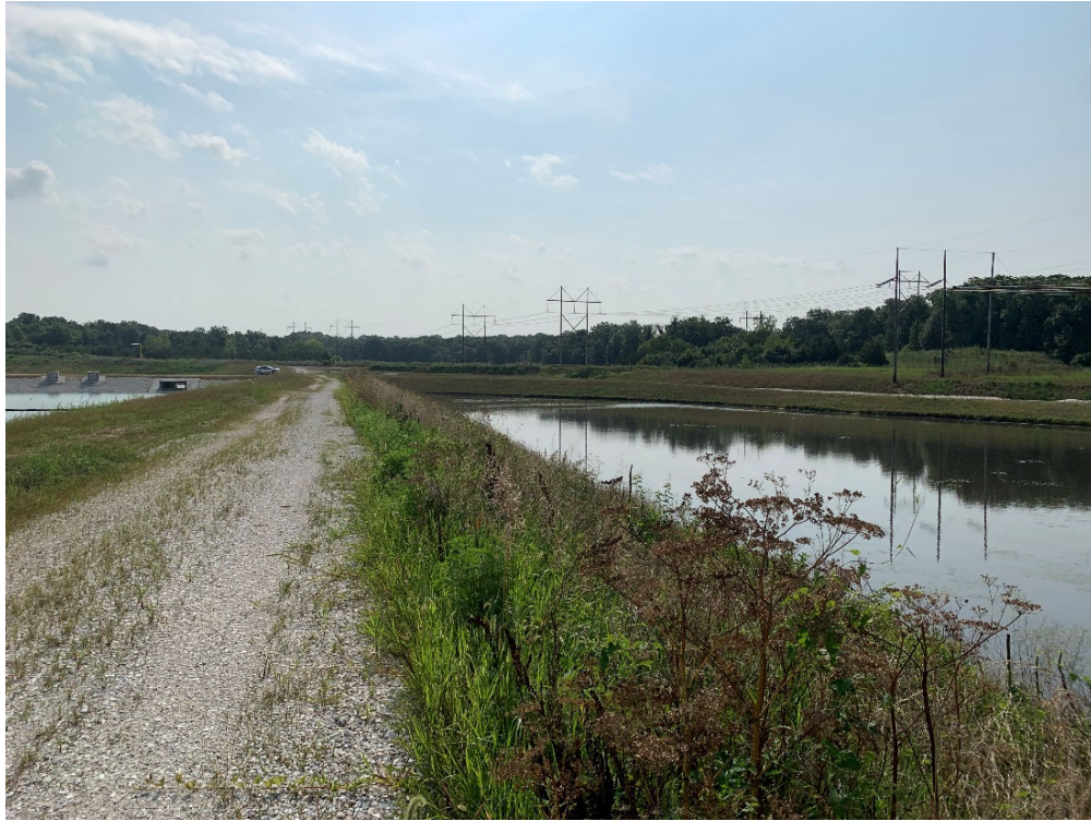
Photo No. 5 Tall vegetation near midpoint of Cell 002 downstream slope
