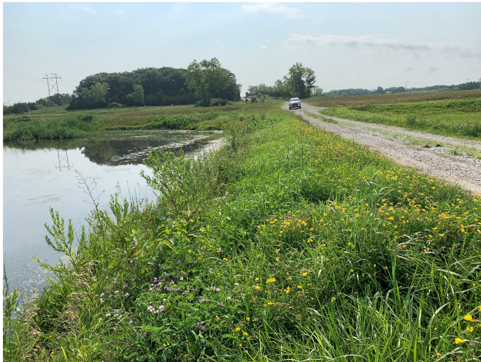
Photo No. 10 Tall vegetation along upstream slope of Cell 003 embankment facing southeast
