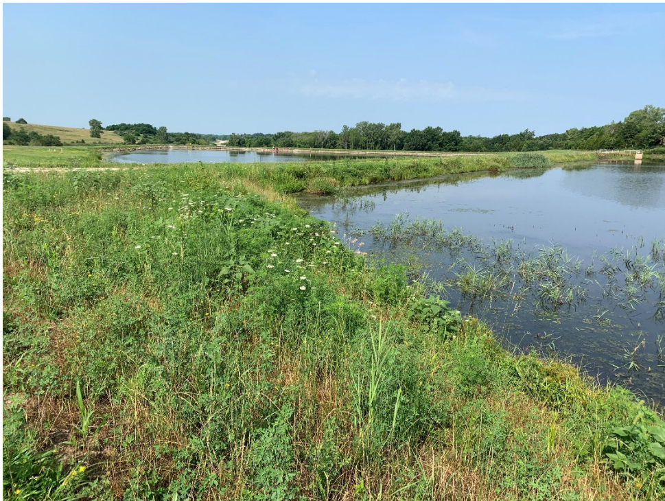
Photo No. 8 Vegetation greater than 1 ft along upstream slope of Cell 003 embankment
