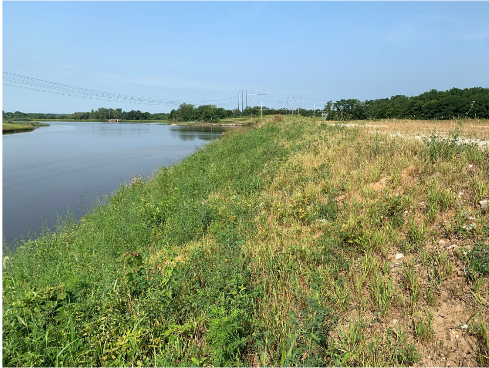
Photo No. 1 Vegetation greater than 1 ft along Cell 002 downstream embankment
