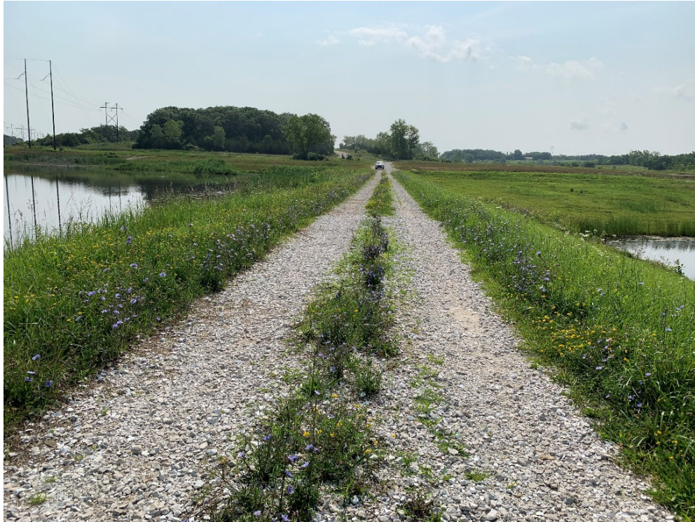
Photo No. 6 Aggregate surface atop Cell 003 embankment crest facing east
