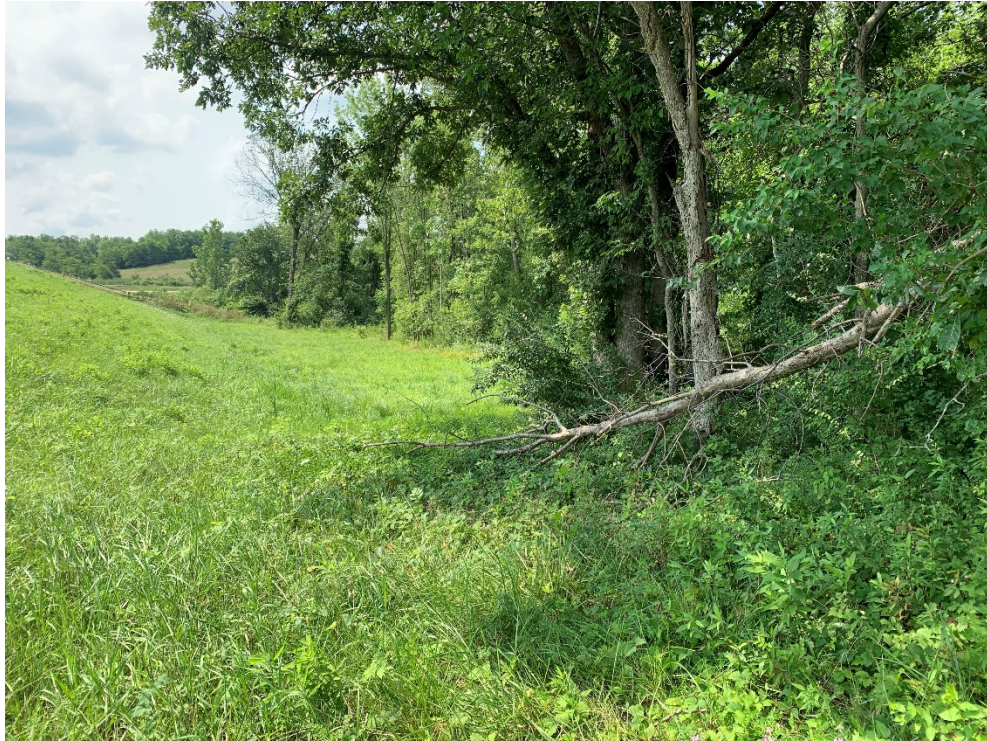
Photo No. 29 Woody vegetation near toe of slope at Cell 004 west embankment
