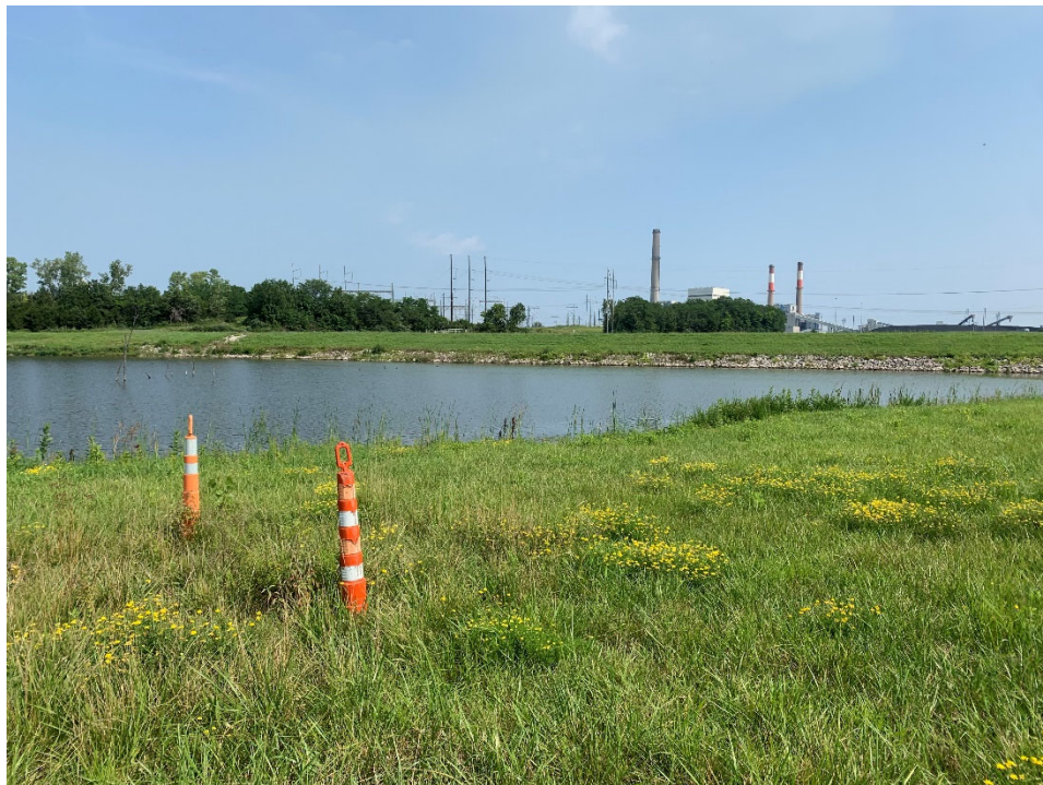
Photo No. 12 Vegetation greater than 1 ft along east embankment Overview of Cell 003 embankment in background
