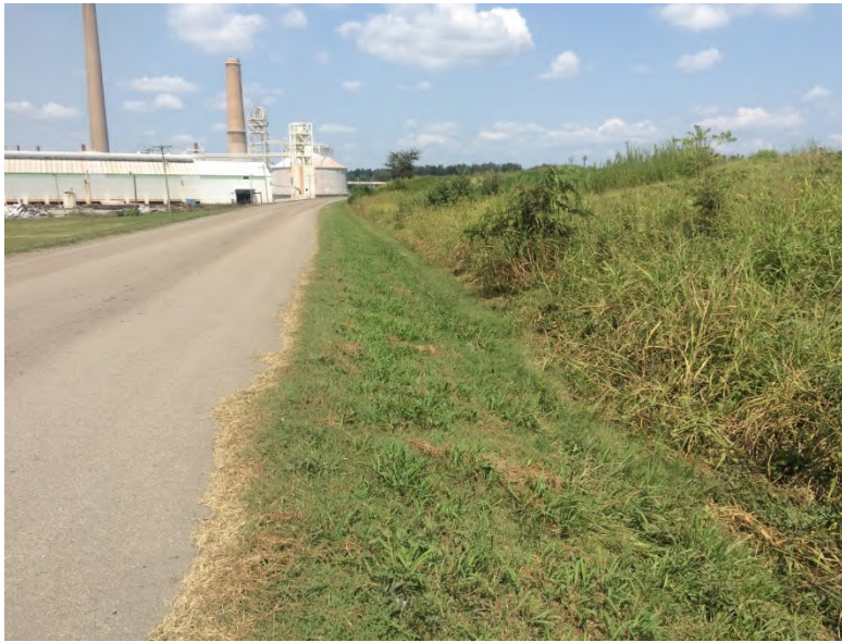
Photograph No. 13 Pond 003 Upstream slope on western embankment Note vegetation growing on Ash stockpiled above water level to the right.
