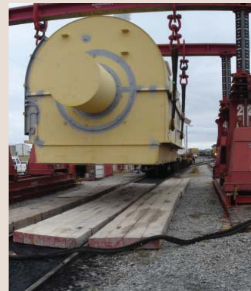
A 718,000-pound generator is lifted from rail sidings for placement on a trailer with 16 rows of 16 wheels, 256 in total, for transport to Associated's Chouteau 2 Power Plant under construction in Pryor, Okla.
