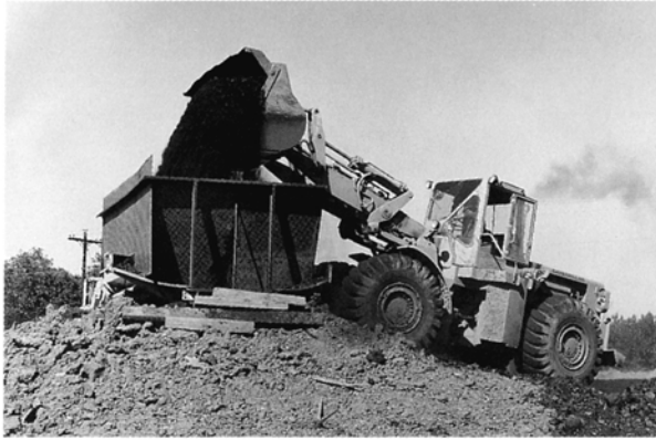
A front-end loader dumps coal from the new Prairie Hill Mine into a temporary coal hopper at Thomas Hill set up to handle coal from Peabody brought over in trucks and dumped in piles.
