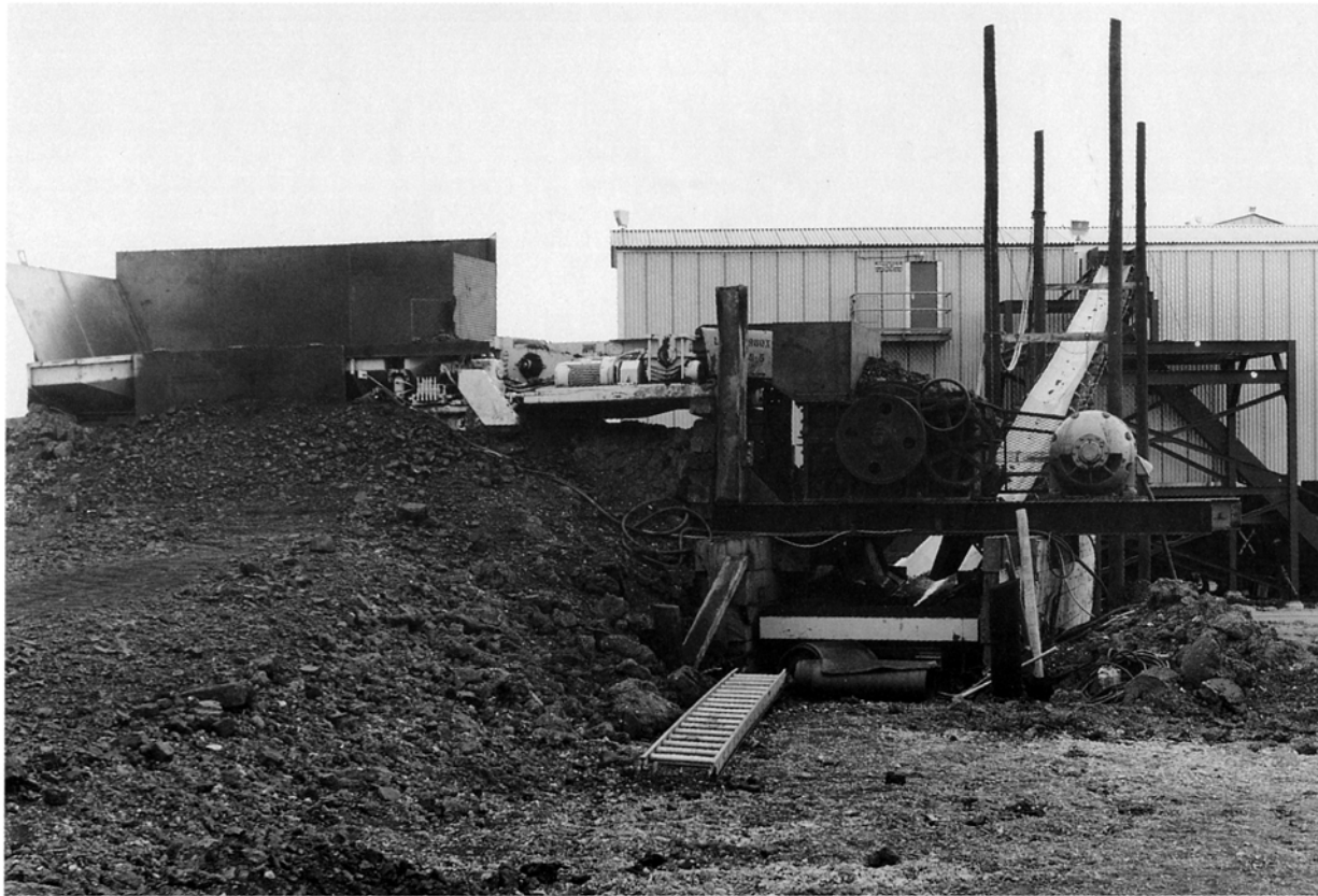
Trucks haul coal from a new Peabody mine, Prairie Hill, adjacent to Thomas Hill Power Plant, and dump it near a temporary conveyor set up beside the car shaker. A front-end loader fills the hopper on the left which diverts coal to the conveyor, right. The conveyor enters the top of the car shaker on this north side and a chute transfers coal into the track hopper where bottom-dump train cars ordinarily unload coal for units 1 and 2.
