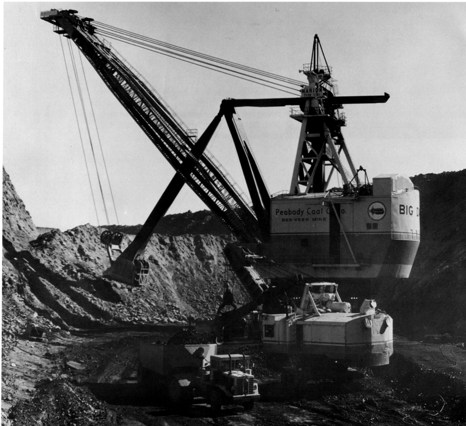
Peabody Coal Co.'s Big David shovel removes dirt and rock covering the coal seam in the Bee Veer Mine near Bevier which supplies coal, delivered by rail, to Thomas Hill Power Plant in 1966.
