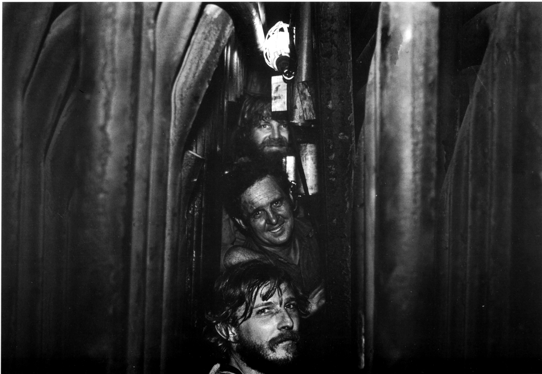
To access damaged boiler tubes in the superheater section of New Madrid's Unit 1, workers pry apart suspended tube sections, creating just enough space to work. Pictured in August 1979 are, from front, mechanics Gilbert Pritchett, Billy Borders and Neal Houseman.
