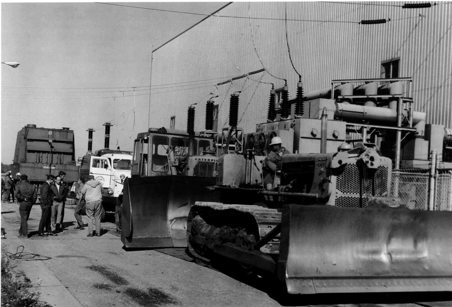
Thomas Hill and Northeast employees work several days to move a step-up transformer away from the plant and prepare it for shipment to the manufacturer for repairs. Despite their efforts, the 162 tons of dead weight will not budge using a winch truck, pulleys and a Caterpillar dozer. Finally, the coal yard dozer is used to load the transformer onto a specially designed railroad car Oct. 30, 1970. Driving the dozer is Al Rustemeyer. Also pictured are Bill Muckelrath, second from left; Paul Smith, second from right; and Enis Colley, far right.
