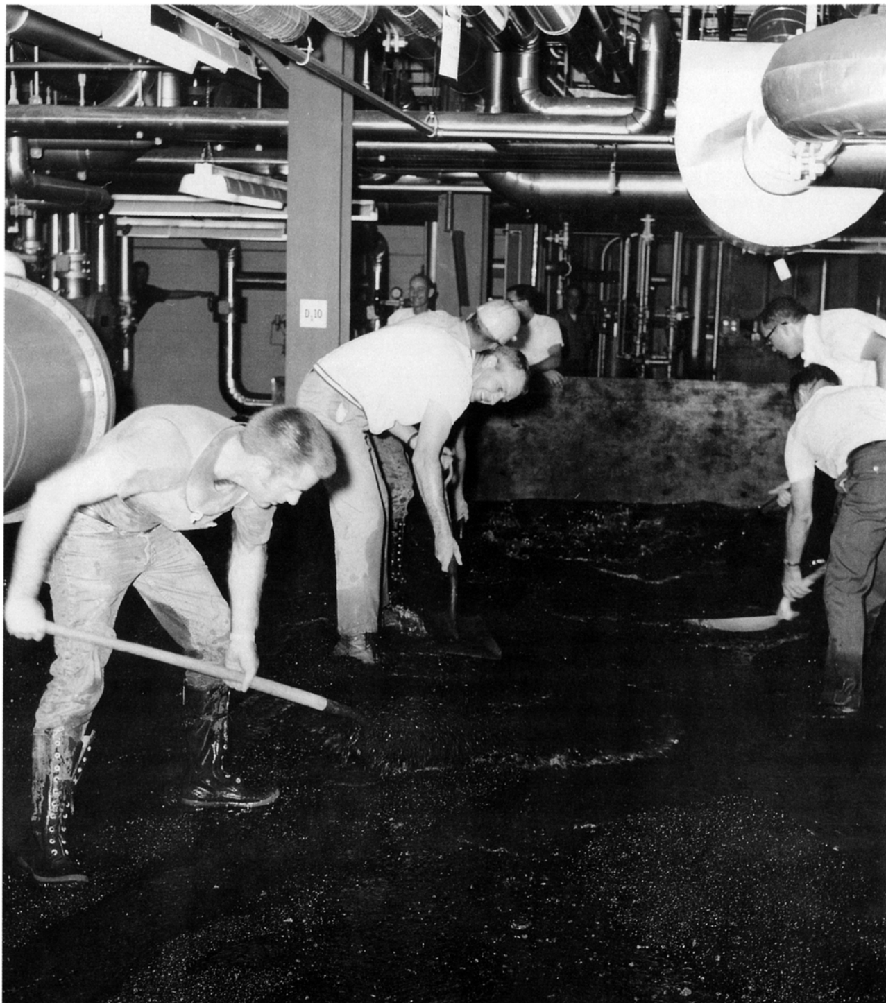
Trying to keep Unit 2 on-line, employees shovel slag off the basement floor at Thomas Hill. Slag tanks had reached capacity, forcing a decision to shut down the unit or empty the tanks. To avoid taking the unit out of service in September 1970, slag is sluiced directly onto the basement floor instead of being diverted through long pipelines to the slag ponds. Shoveling, on left, are Jerry Teter and Ed Vroom. On the right are Paul Smith and Bill Muckelrath. In the background, George Walbrink, left, and Jesse Burton watch.
