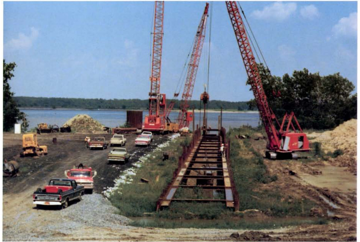
With the Mississippi River as a backdrop, New Madrid Unit 2 construction continues with this coffer dam July 10, 1974.
