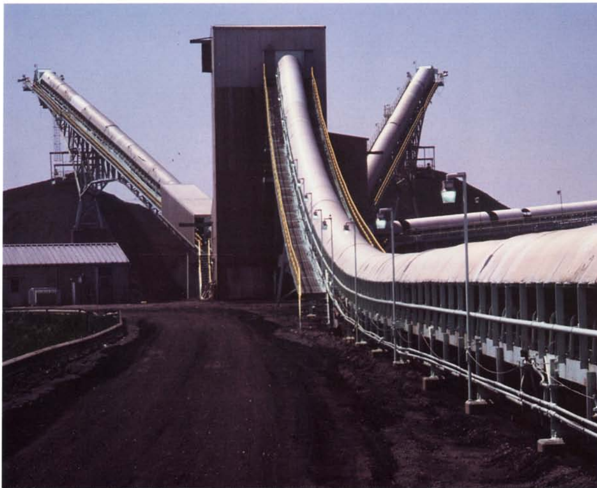
An elaborate system of conveyors delivers southern Illinois coal from barges on the Mississippi River to the New Madrid Power Plant coal yard. At full production, New Madrid burns 12,000 tons of this high-sulfur coal each day during the 1980s.
