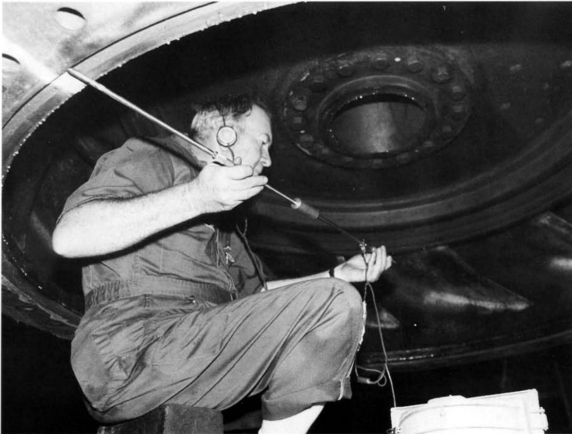
To diagnose problems with a circulating water pump, machinist J.B. Perry listens through headphones attached to a monitoring device.
