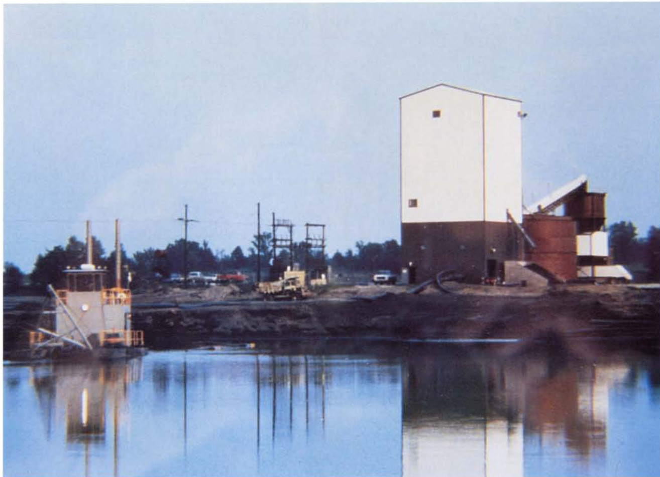
The U.S. Department of the Interior recognizes Associated with one of nine 1989 Excellence in Surface Coal Mining and Reclamation Awards for the Bee Veer preparation plant. The plant processes coal slurry from an old coal washing plant to extract fine coal particles to burn at Thomas Hill Power Division, turning a reclamation liability into a coal resource.
