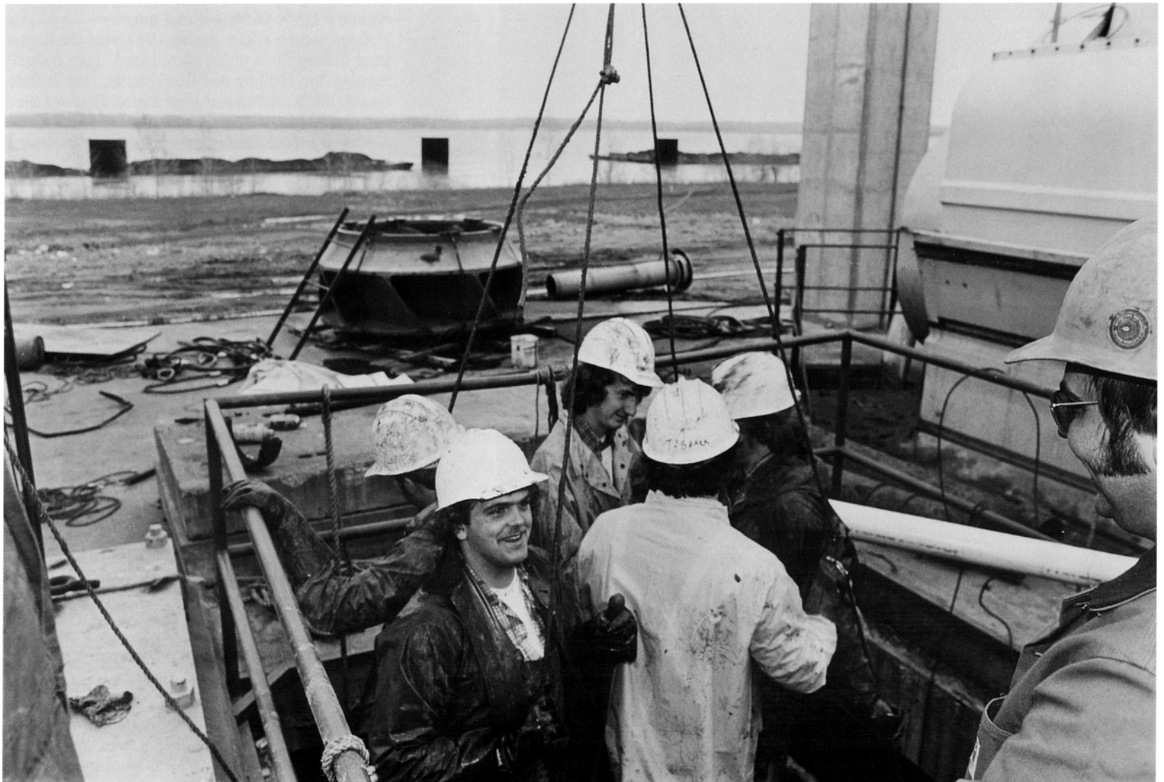
To clean debris from New Madrid Unit 1's circulating water pit, a group of workers is lowered in a basket. Among them is Elmer Coffey, center back. Tommy Sides, far right, watches them descend.
