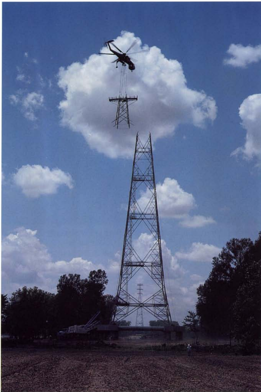
A helicopter lowers a section of tower in 1993 to help complete a transmission project connecting Associated with the Tennessee Valley Authority (TVA). Associated is the first new party TVA interconnects with since 1968.
