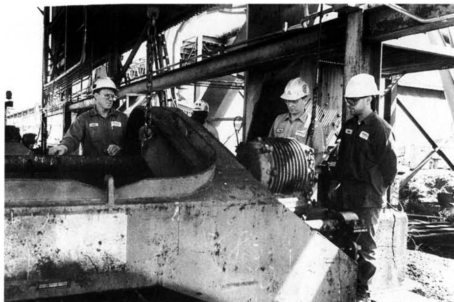
Thomas Hill Power Division employees, from left, Paul McCloud, Greg Jacobs, Tony Joseph and Jim Kraft hoist a shaker used on top of a rail car to unload bottom-dump rail cars in 1994, when Associated is converting its facilities to unload and burn low-sulfur coal.
