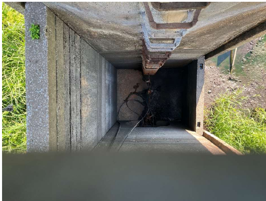
Photo 6: Looking down at the concrete drop inlet tower structure with stop logs at Cell 004
